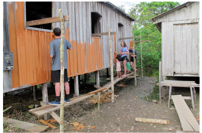
Josh, Lydia, and Netania with some of the local kids painting the church. The homemade scaffolding was made by 'whittling' the ends of 5" logs so that they were 'spear' like and then ramming them into the mud.
